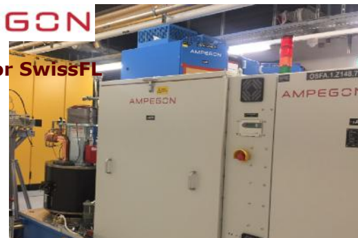
13 modulators (Linac 1, Linac 2)
