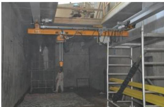
Figure 2: The klystron gallery tunnel with a 3.2 t crane.
