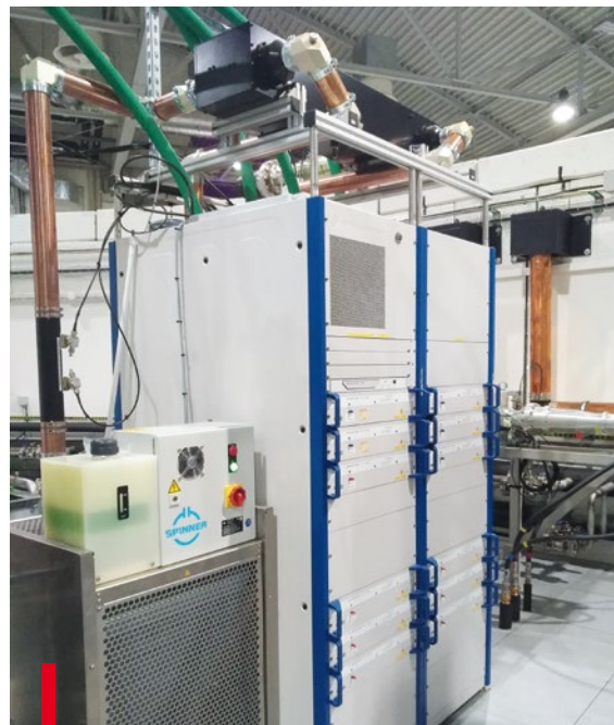
Transmitter THR9 100 MHz 100 MHz Rhode&Schwarz transmitter
